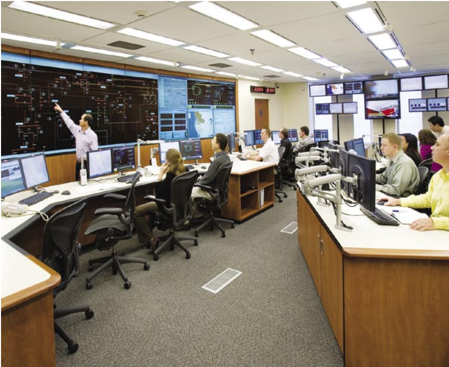
RESEARCHERS at the Pacific Northwest National Laboratory sit in a simulated regional control center and test prototype software that would provide human operators with real-time grid information, necessary to stop a nascent blackout before it expands.
